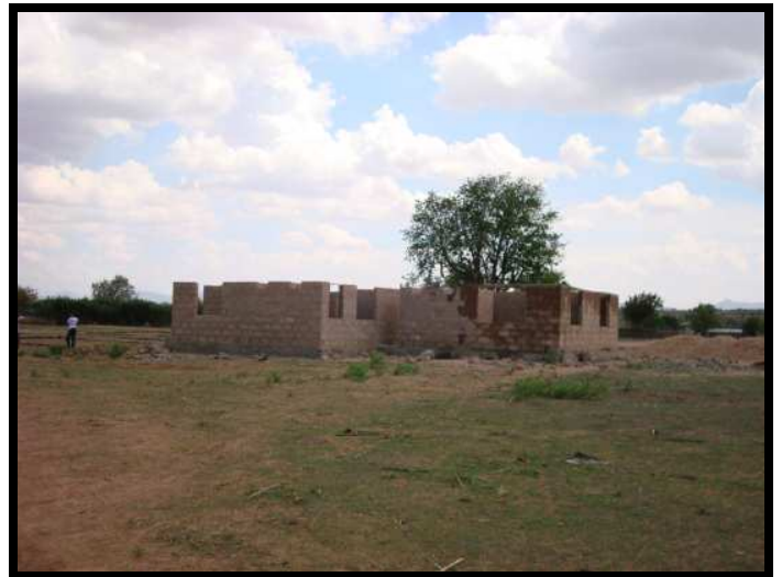
Partly completed 'home' = Children's Home Mahoma Makulu
